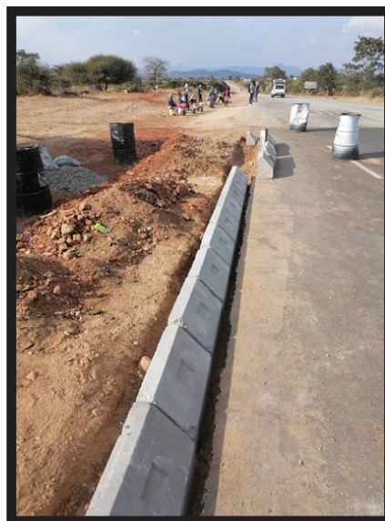
Lining kerb stones at Mhandamabwe intersection.
