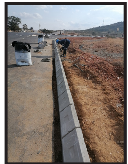
Mhandamabwe intersection last stretch of kerb stones being installed.
