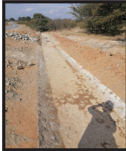
Stone pitching in progress.
